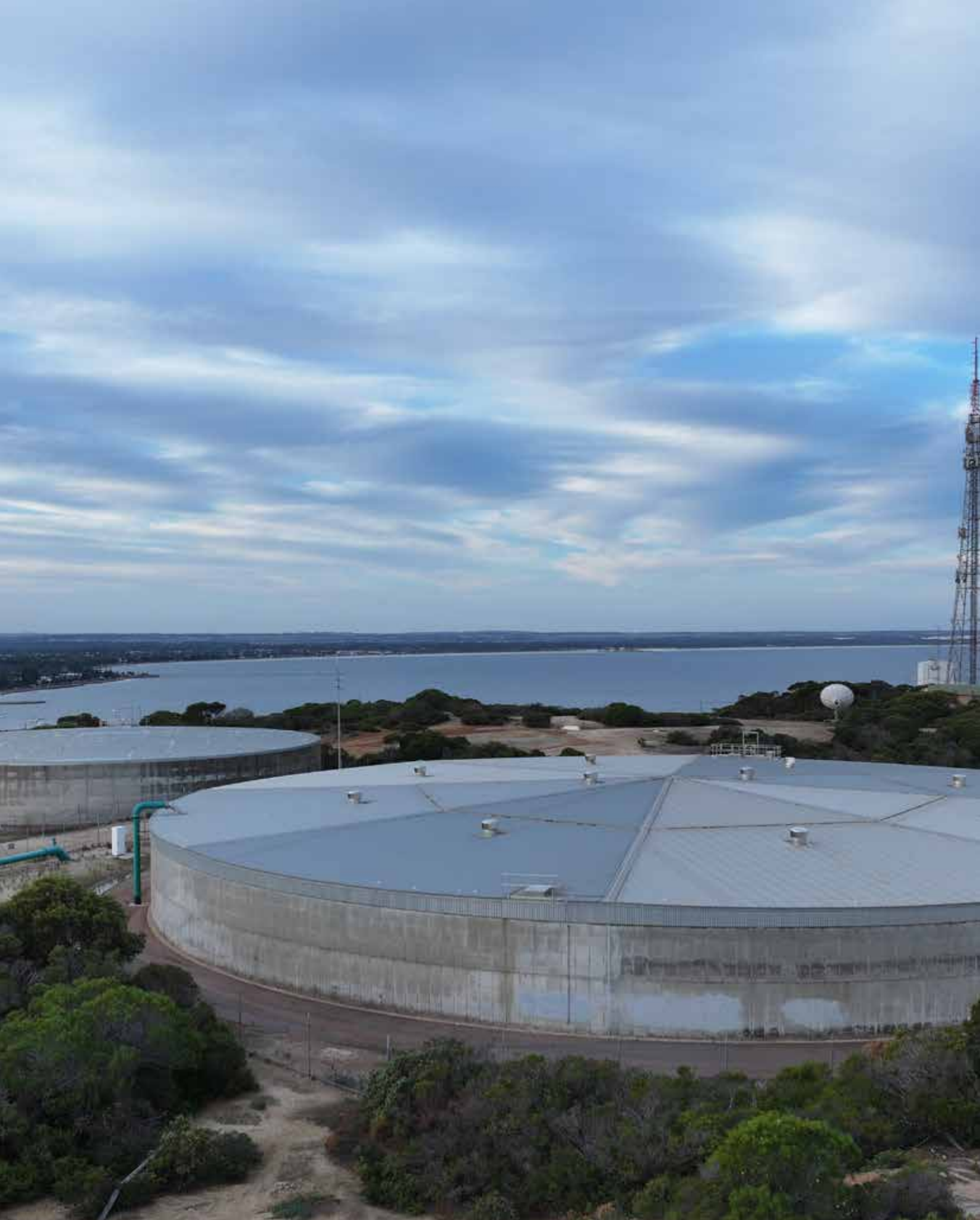
Image: Wireless Hill Water Tank, Esperance
